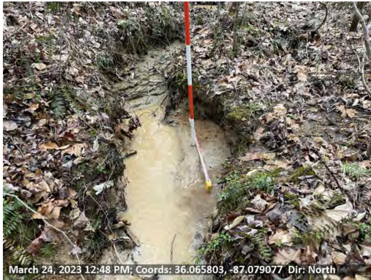
27 View of WWC-18-A proposed sediment removal location on left descending bank, measuring approximately 3'x1', and 3" deep.
