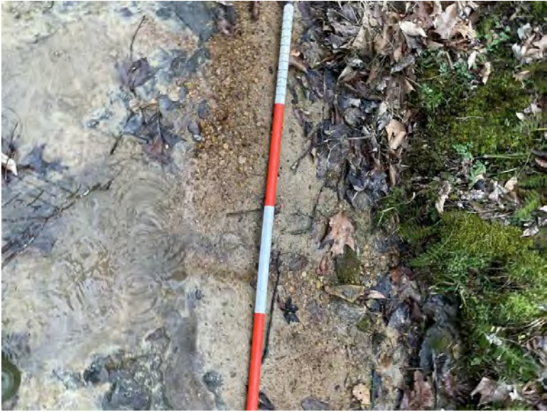
3 View of STR-3-C proposed sediment removal location on the right descending bank measuring approximately 4'x1', and 0.5" deep.
