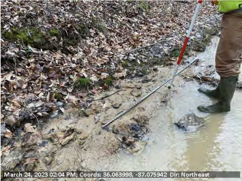
19 View of STR-6-H proposed sediment removal location on left descending bank measuring approximately 5'x2', 0.25" deep.
