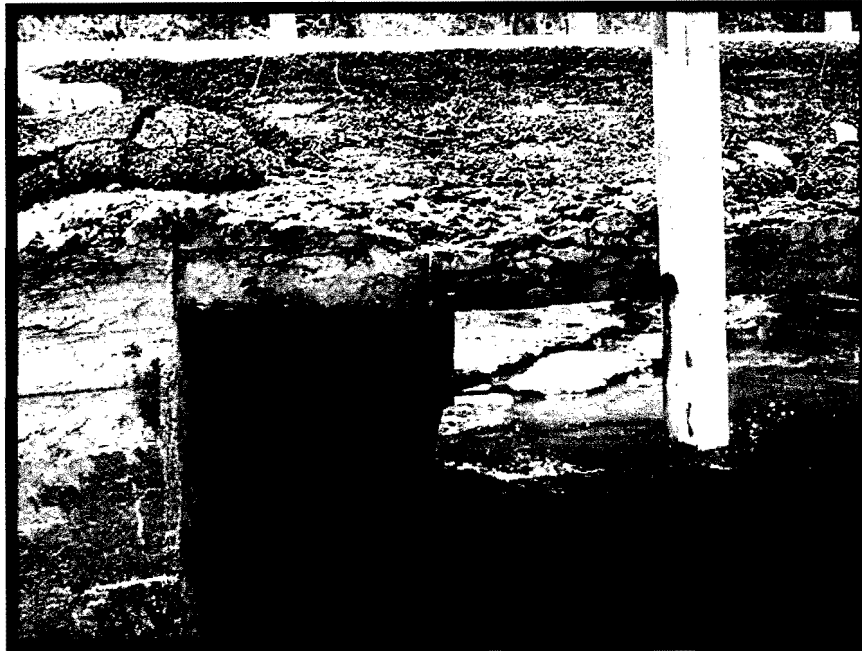
Photo No. 9 – Sag in Bridge Deck
