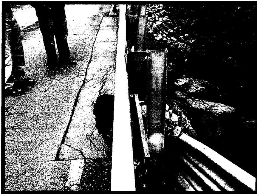
Photo No. 2 – Asphalt Failure
